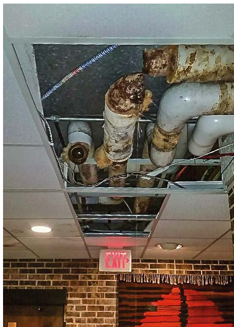
Before: Old piping in the ceiling showing severe corrosion.
