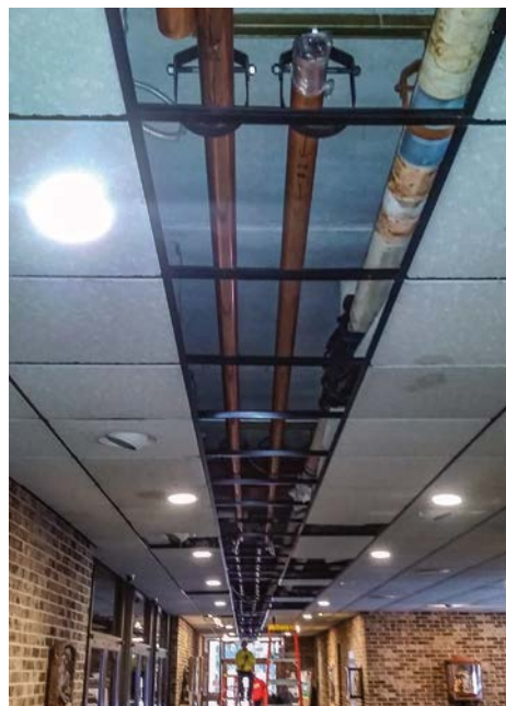
After: New copper piping installed in the ceiling.
