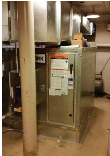
Newly-installed modular air handler.
