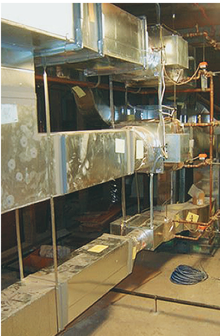
New air ducts and VAVs
