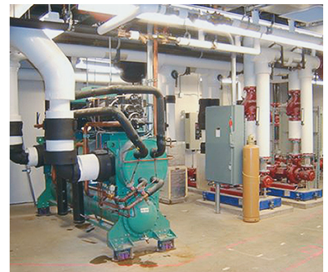
A new chiller and pumps were installed
