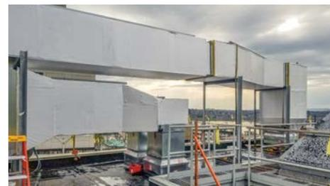
Insulated ductwork installed on the roof.
