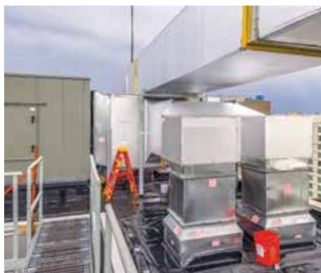
Insulated ductwork tie-ins.
