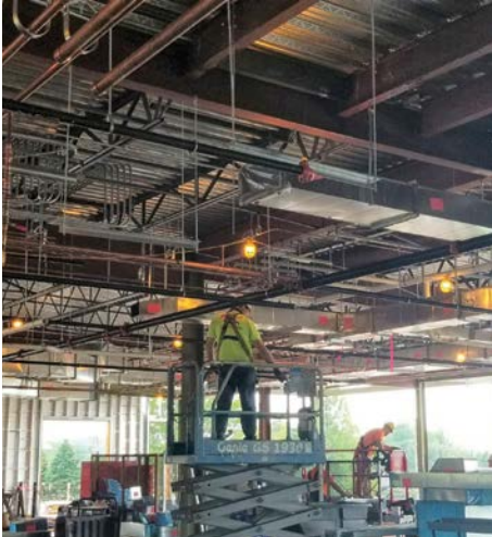
Second floor duct installation
